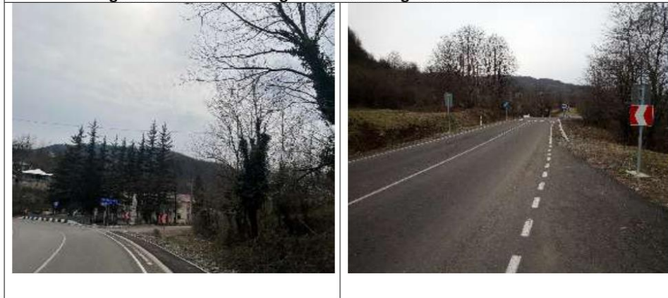
Figures 5 and 6: Road Signs on and along the Lot 1 Road Section
