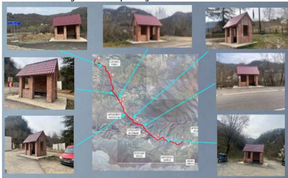
Figure 7. Bus Stops Along the Lot 1 Road Sections
