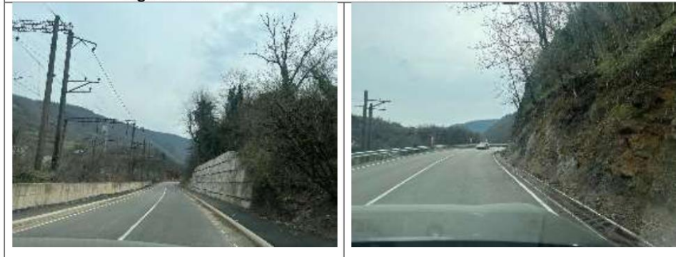
Figures 3 and 4: Road Pavement in the Lot 1 Road Section
